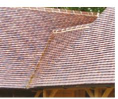
New Machine Made Clay Tile
