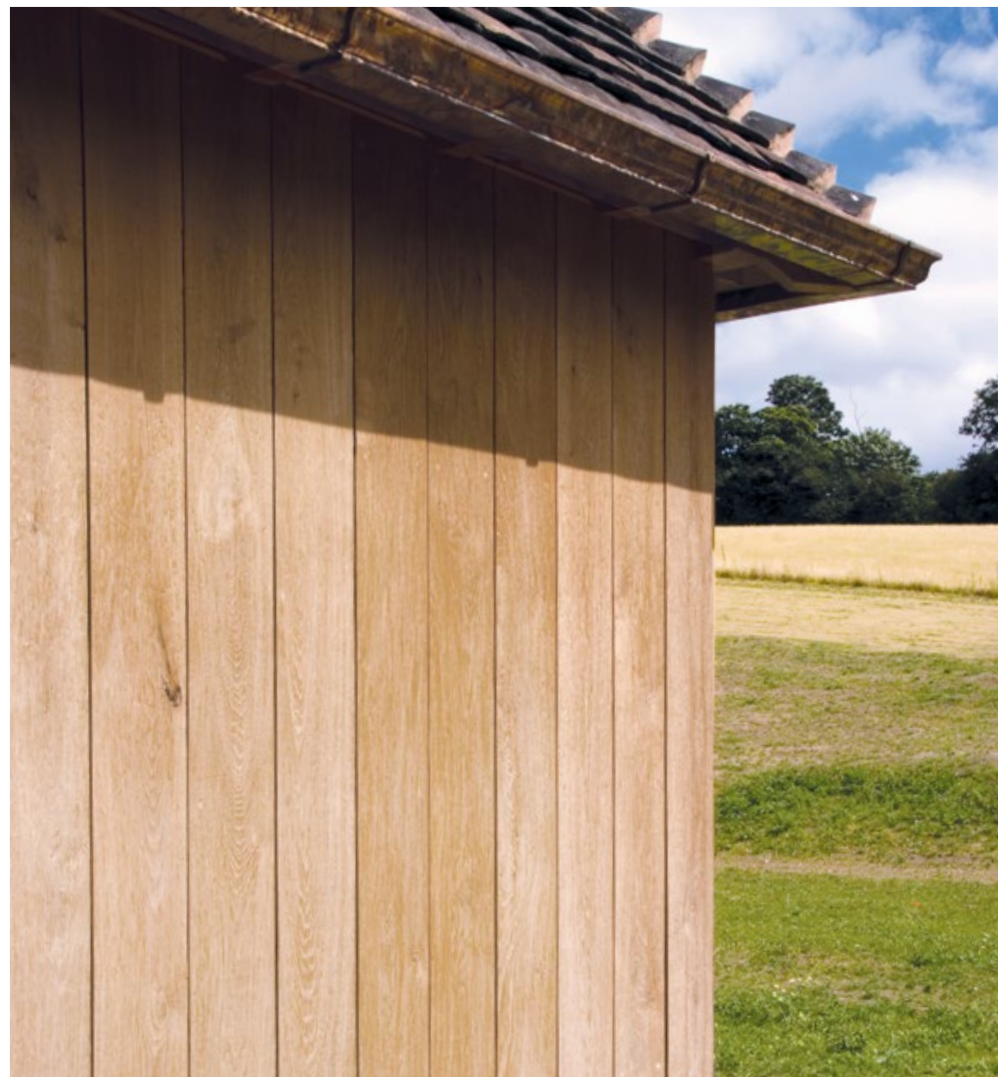
Vertical Oak weatherboard with our gasket detail provides a contemporary choice of finish.
